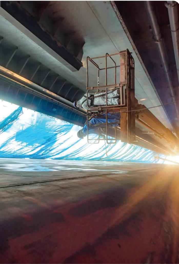
Rigging equipment must be free from defects, fit for purpose, marked to indicate its working load limit, adequately maintained and subject to relevant legal requirements for inspection with valid certification must be available upon request.
