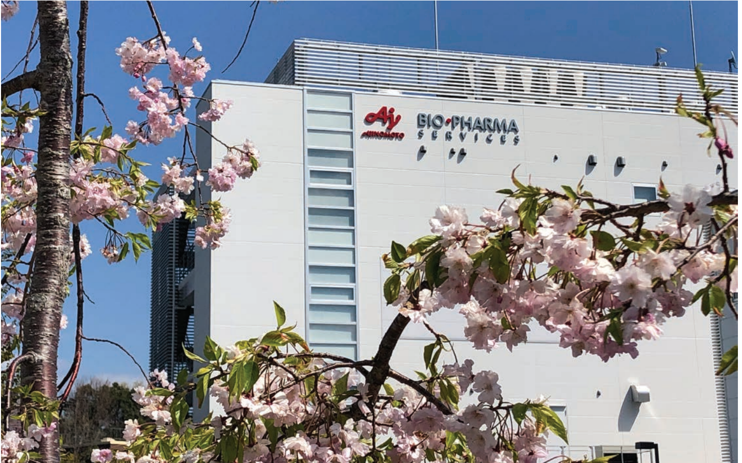
Ajinomoto Bio-Pharma Services Oligonucleotide API Manufacturing Center at the Osaka, Japan campus.
